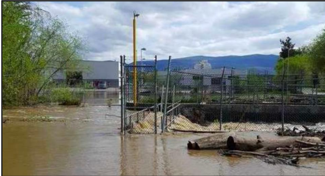
Figure 9 – Mill Creek Diversion Gate during 2017 freshet (photo: Infotel)
